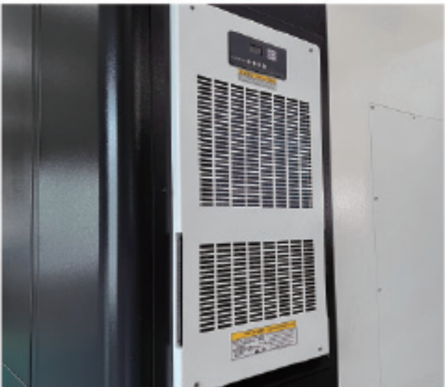
Electric cabinet cooling air conditioner
